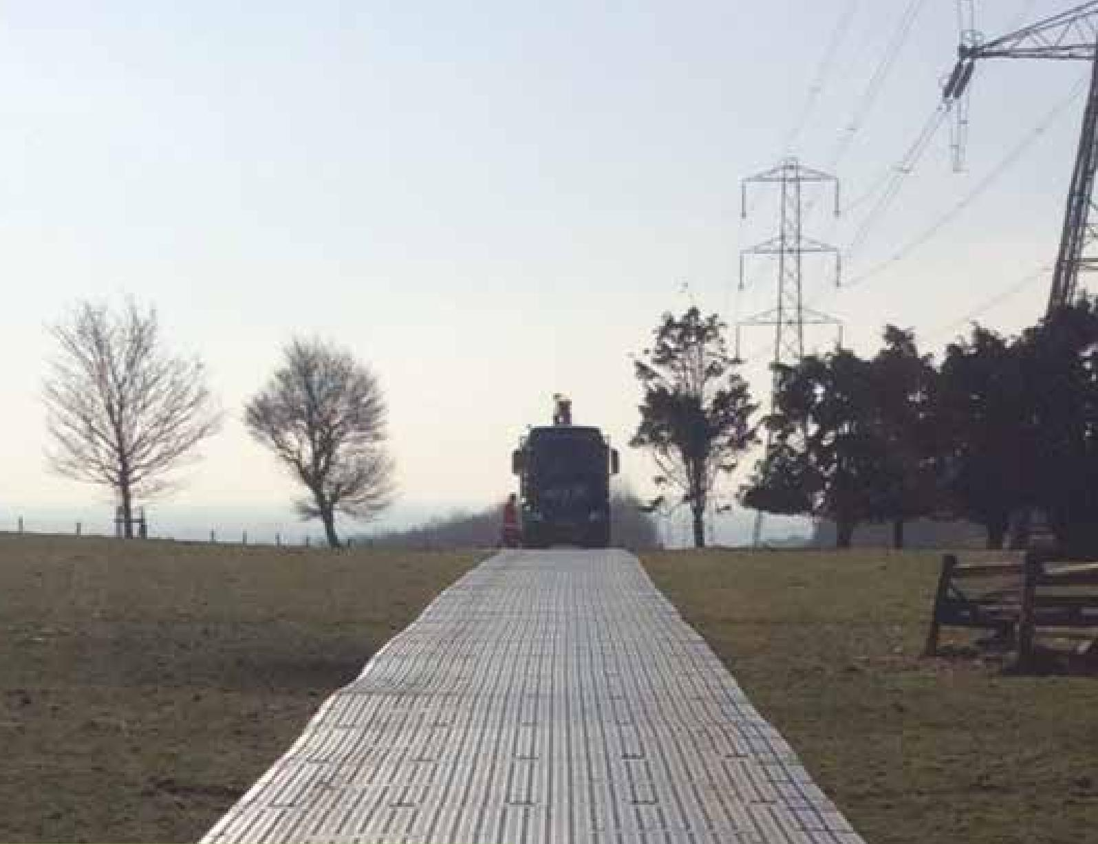
TuffTrak® offers a full range of market leading composite ground protection mats delivering a safer work environment for temporary access roadways, trackways, and working platforms.
